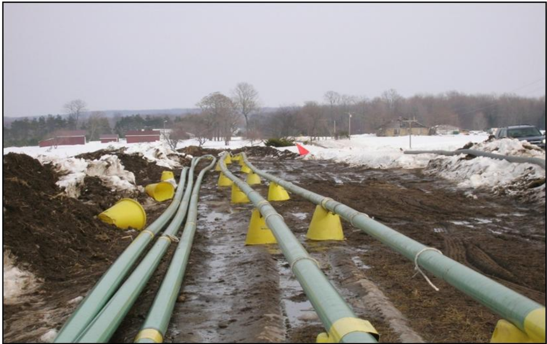
Figure 9 - New Albany Shale Gas and Water Lines Prior to Burial 4
