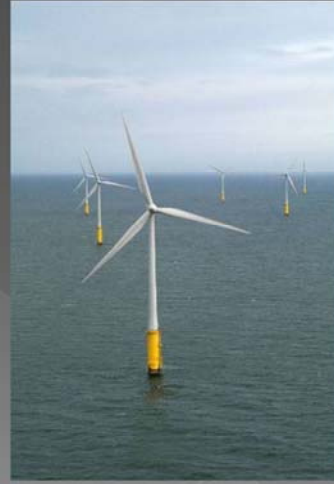
V80-2.0 MW, North Hoyle, UK
