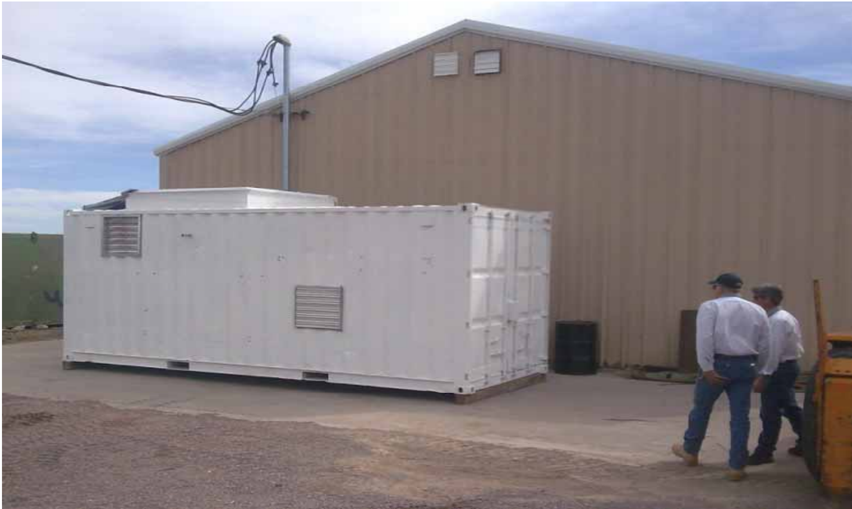
Trailer holding the water purification unit
