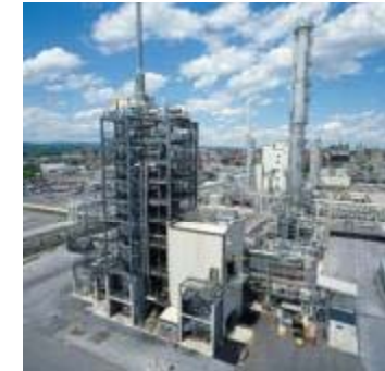
Commercial Gasification Plant
