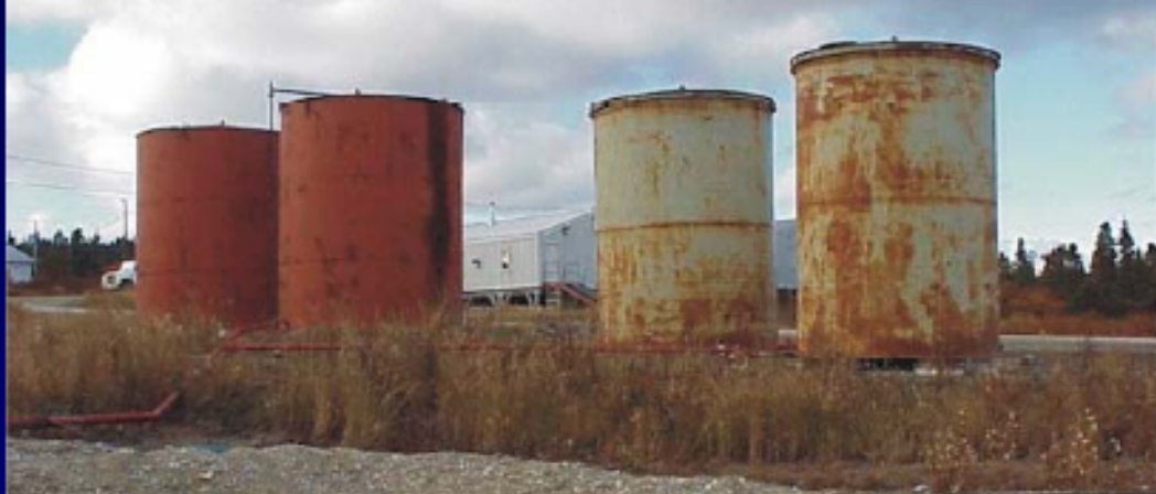
Typical view before replacing and upgrading tank farms in rural Alaska.
